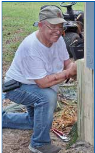
NIC disaster response workers built a temporary electrical service pole.
