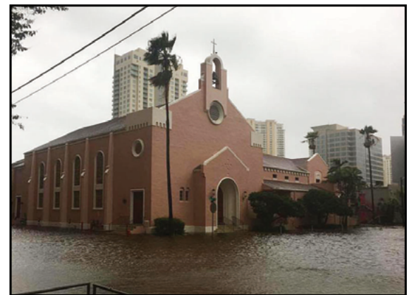
First United Methodist Church in Fort Lauderdale, Fla., is surrounded by floodwaters following Hurricane Irma. Photo courtesy of First United Methodist Church in Fort Lauderdale via Facebook.
