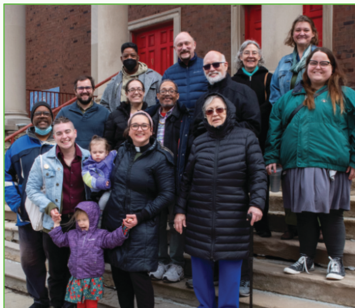
Current members of United Church of Rogers Park stand cautiously on the deteriorating front steps leading to the church's main entrance. A capital campaign will help create a state-of-the-art front entrance and make the church more accessible and welcoming to all.
