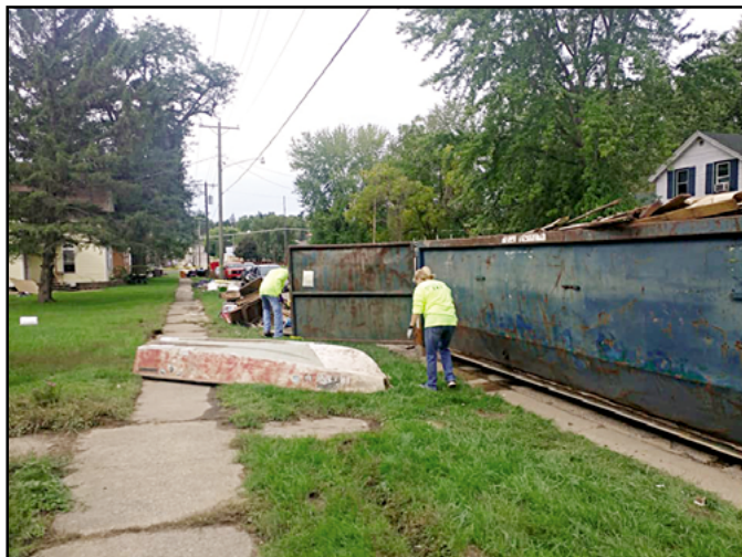
The crew helps fill several large dumpsters stacked along the curb with debris.
